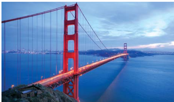
Golden Gate Bridge.
