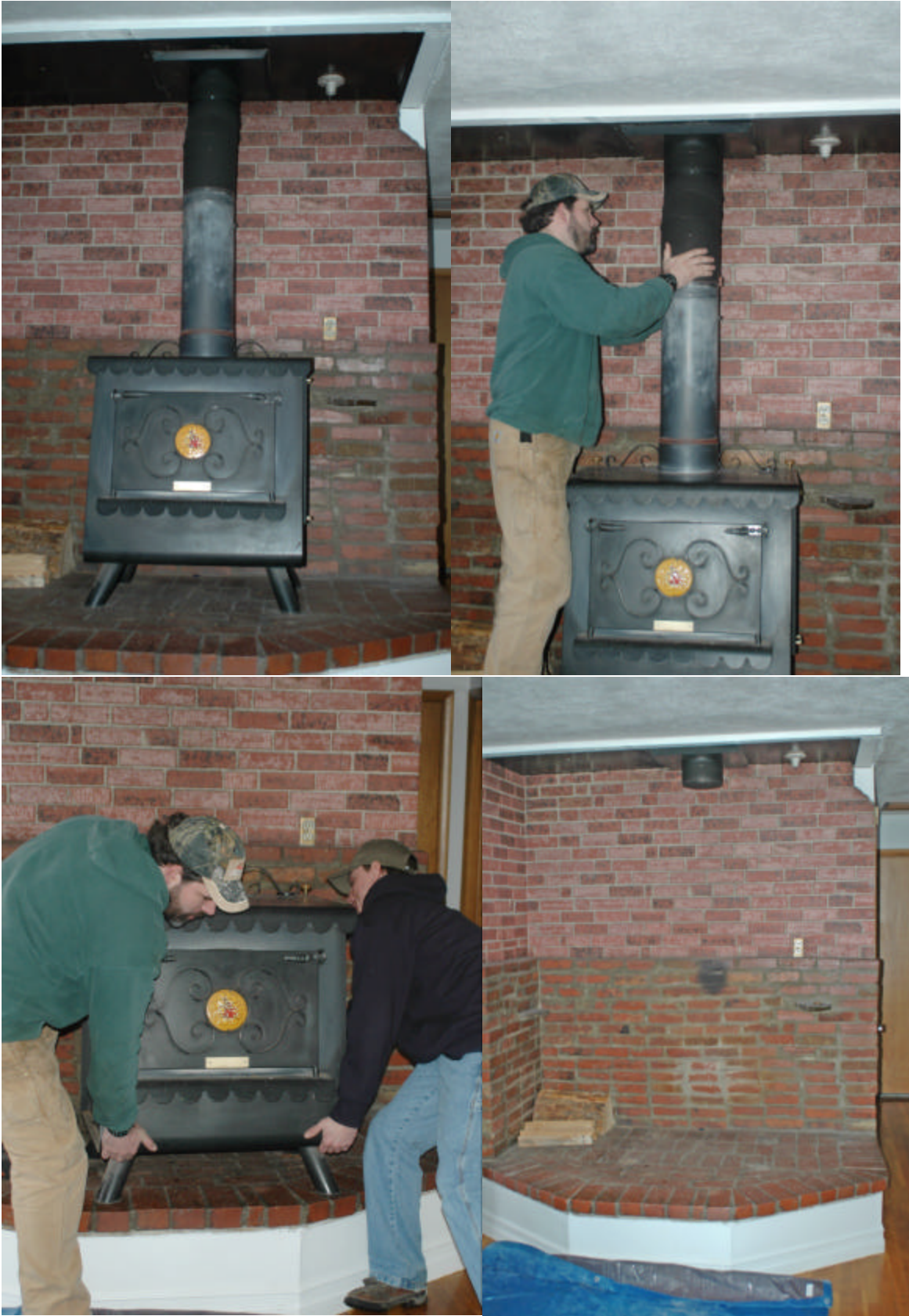
Figure 4. Photographic Documentation of Typical Woodstove Changeout
